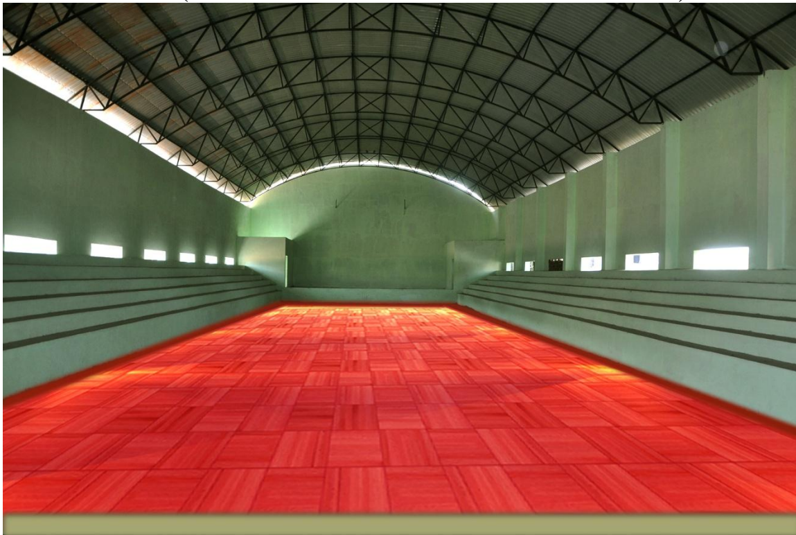
(INTERIOR VIE OF THE INDOOR STADIUM)
